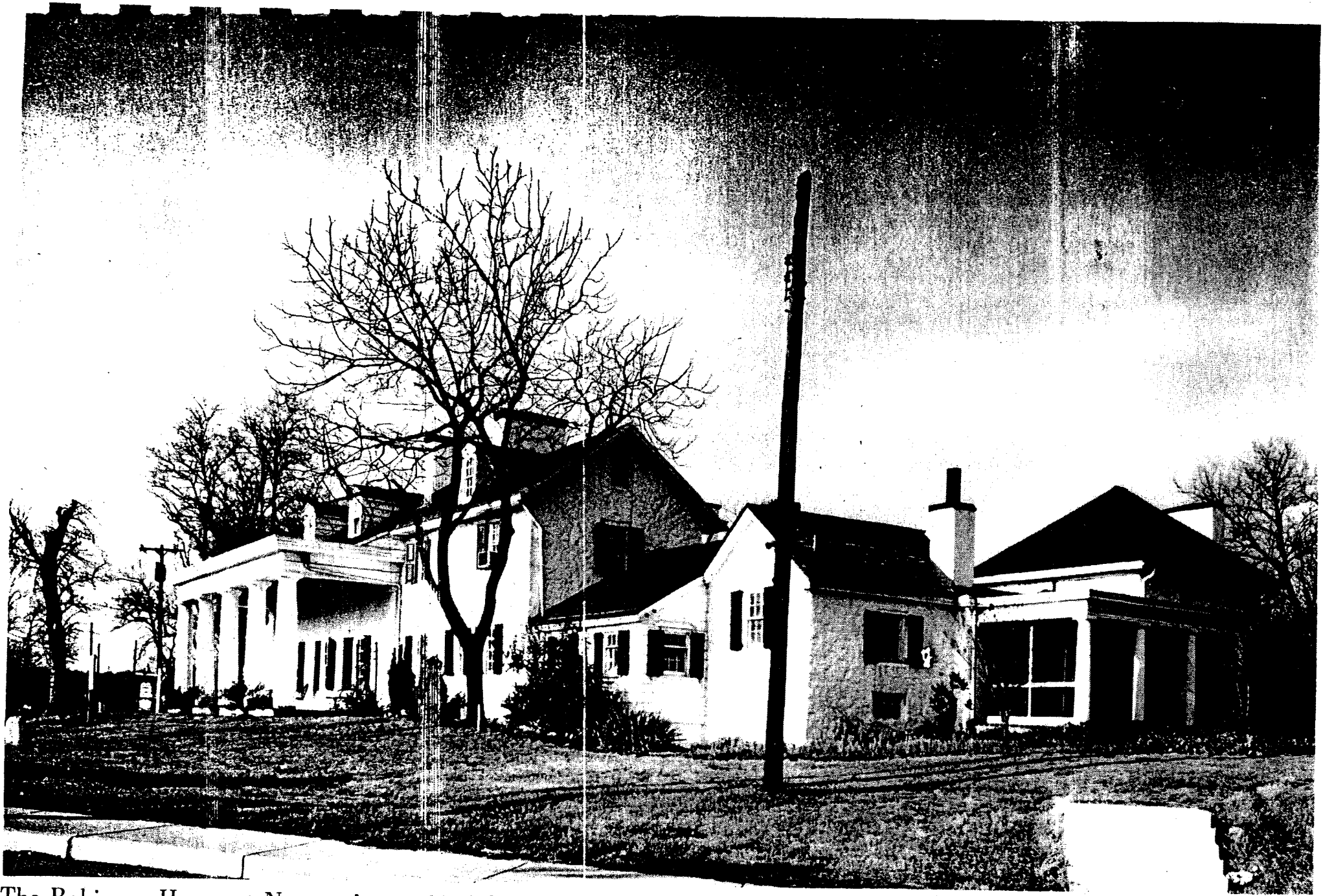
The Robinson House at Naaman's, north of Claymont, west front view.
